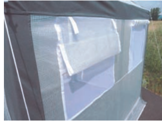
Adjustable, screened windows for cross ventilation control
